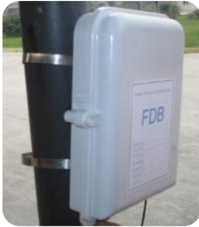
FTTH termination box on the pole
